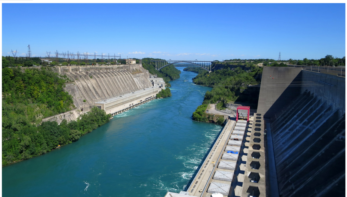
The Robert Moses Niagara Power Plant in New York.
